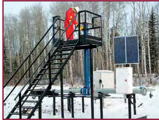
Alberta, Canada 6 inch 600 ANSI, eleven pig capacity Self-contained solar electrically actuated
